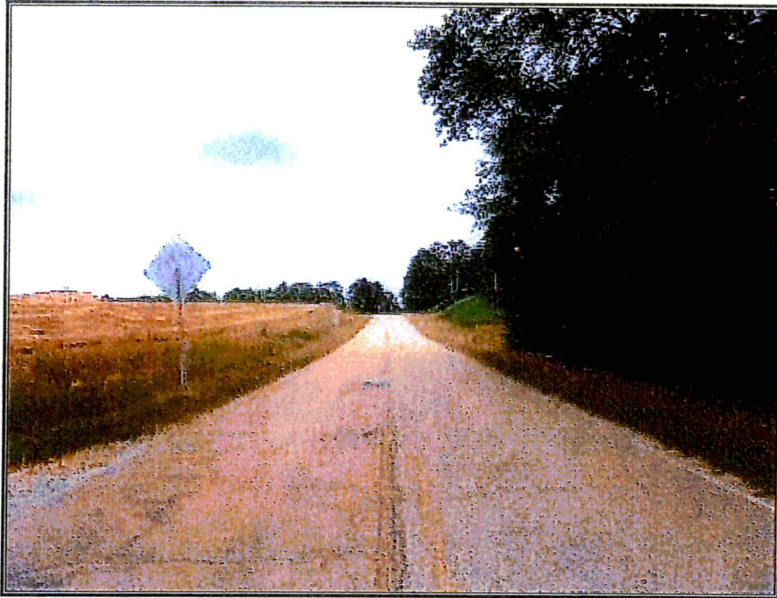
Viewing southwest along Sulphur Springs Rd. in front of subject
